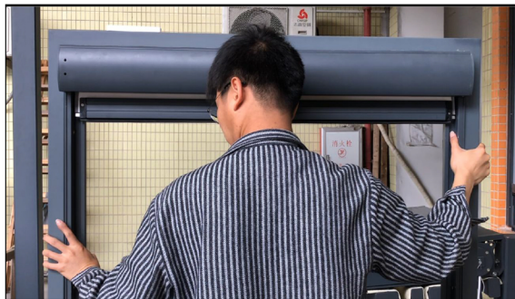
4. Put the rolling curtain into the installation position, observe whether the rolling curtain matches the installation position, and measure whether the diagonal length on both sides is consistent?
